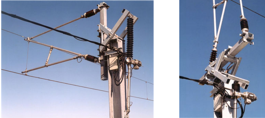
Figure 7.6: Picture of a Kippfahrleitung mast in down and up position
